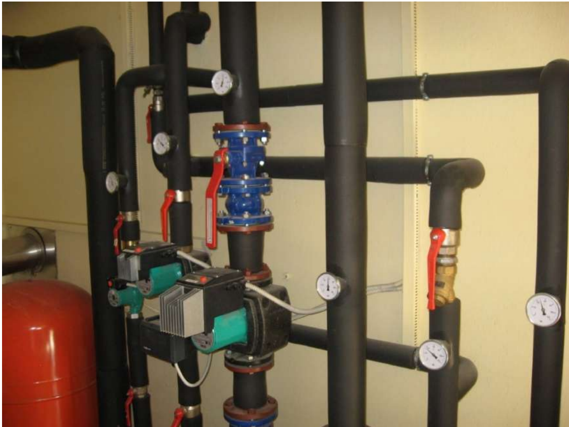
Boiler room, distribution/heating branches (building A)
