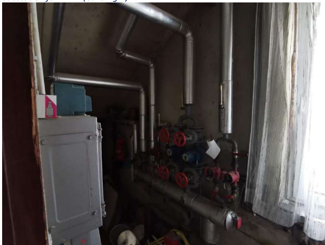
Heating substation for DHW (building B)
