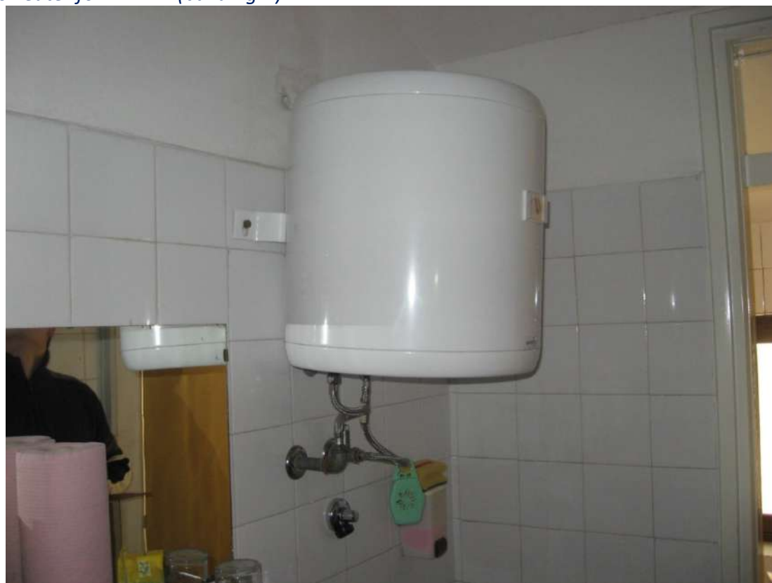
Electric heater for DHW 2 (building A)
