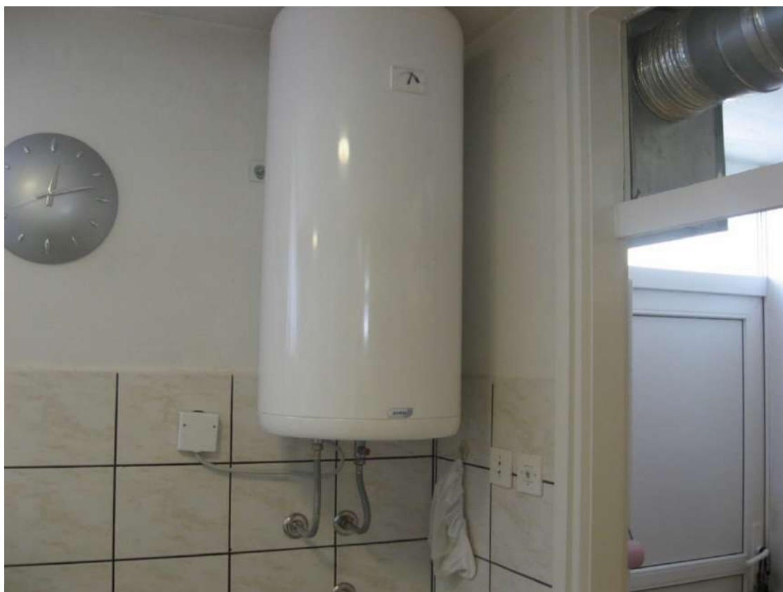
Electric heater for DHW 2 (building A)
