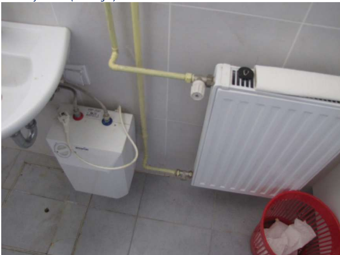
Electric heater for DHW (building A)
